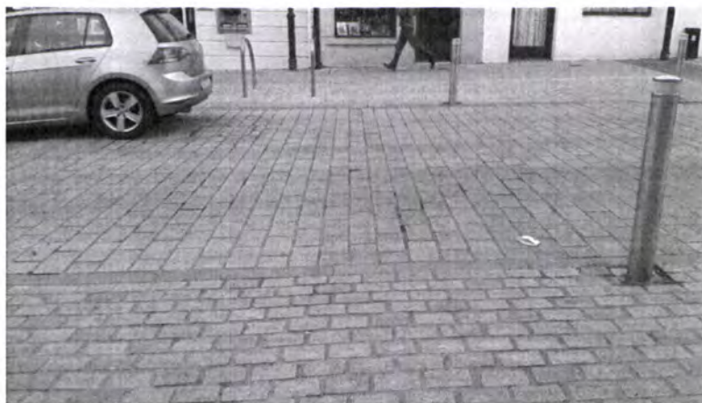
Attractive use of high quality granite used in traffic calming ramps
